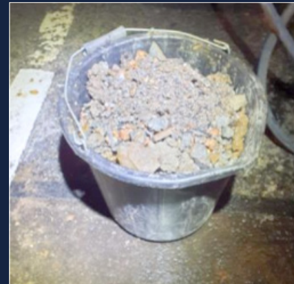
DURING, RUBBLE REMOVED
